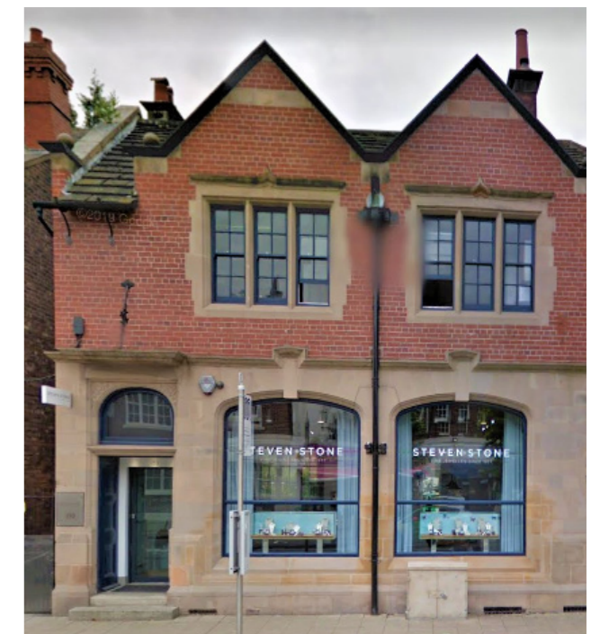
In some cases, buildings that were not traditionally shops will not incorporate a fascia in their design. Well proportioned lettering or signage should be applied directly onto the window
